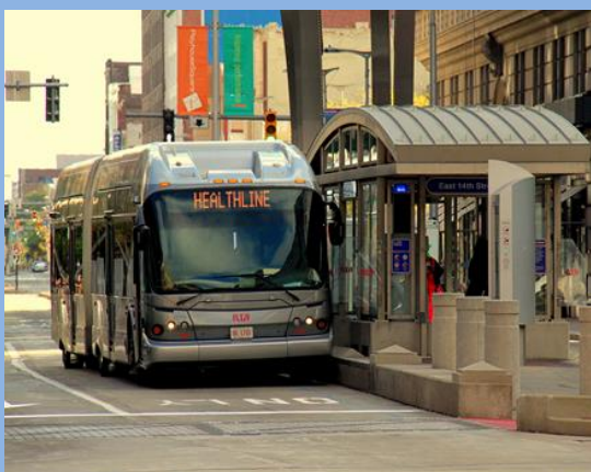
Health Line, Cleveland, OH Dedicated BRT in median--doors on both sides of bus Local example: University of Minnesota transitway
